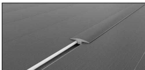
For rooms less than 25 ft (7.6 m) long or wide, leave an expansion gap of 3/8" (10 mm).
