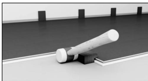
Use a pull bar to install the last plank in a row. Place one end of the pull bar between the wall and the plank and gently tap the other end of the pull bar.
